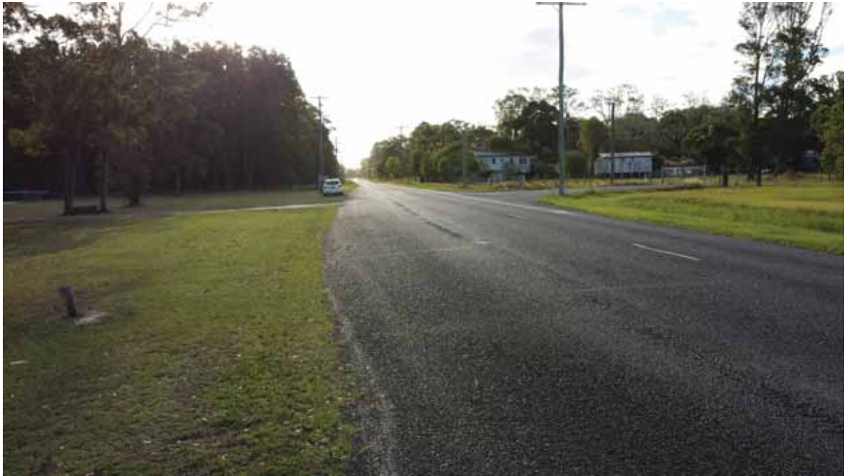
Figure 2 Existing Site Access, looking west
