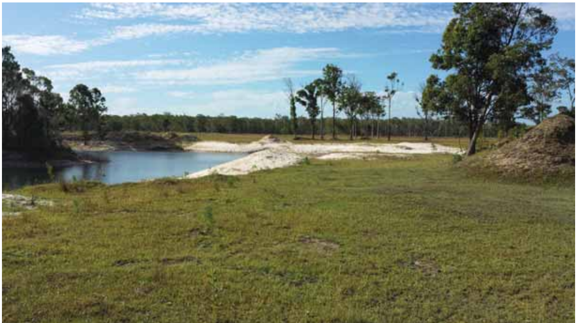
Figure 5-22 View of existing dam and proposed quarry expansion area from the southern portion of the site, adjacent to R8, looking north
